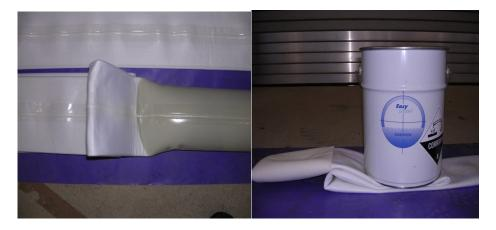
After filling, impregnation/calibration must be carried out immediately to distribute the resin quantities as quickly as possible.
