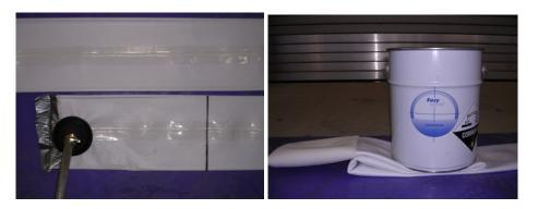
The impregnation process must be stopped at a safe distance in front of the suction cup and the suction cup removed.
