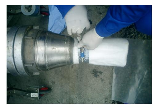
Make sure that the connections are airtight. The mounting window of the inversion drum must also be tightly closed.
