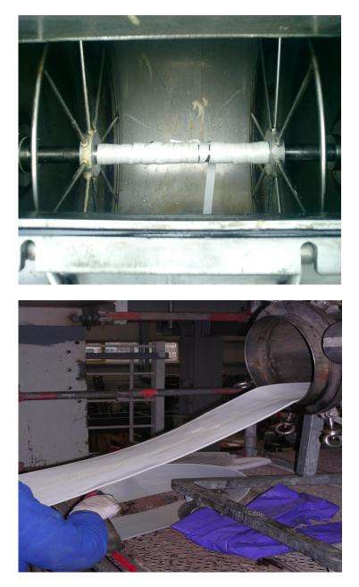
At ambient temperatures above +25  $^{\circ}$ C, the liner must be kept cool (e.g. in a water bath) and the inversion drum must be cooled with cold water (e.g. from the hydrant).
