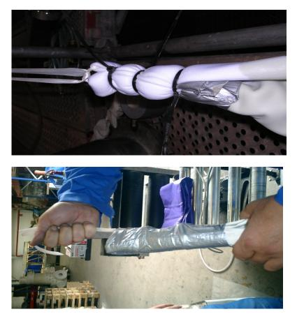
The control tape/webbing in the inversion drum must be wound up tightly. Now the liner can be wound up on the shaft as well. Do not forget to lubricate the EasyLiner system while it is being wound up. Commercially available sponges or a spray bottle are suitable for this. Wetting both sides of the liner is very important. The lubricant ensures good sliding during inversion.
